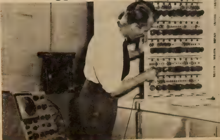
Here is an insight into the electrical and mechanical design of the computer and the accessibility of the components. Components are mounted on chassis fixed to hinged
